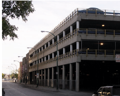
West Facade of the Winnipeg Greyhound Bus Depot Along Balmoral Street
