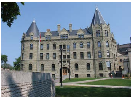
Exterior View of Wesley Hall
