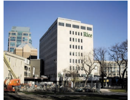
West Facade of the 491 Portage Avenue Complex Along Balmoral Street
