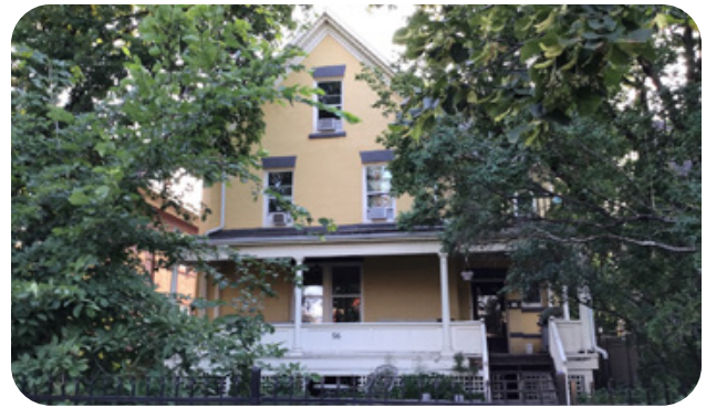
Commonground housing cooperative
