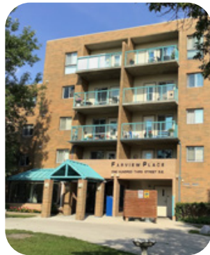
Fairview Place Housing Cooperative, Teulon
